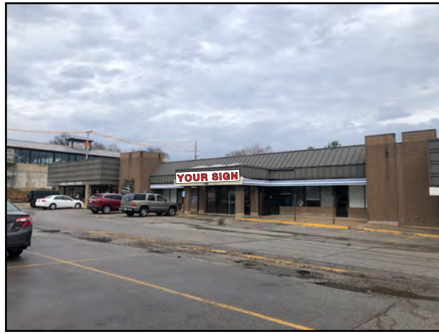
FORMER MEDICAL OFFICE
